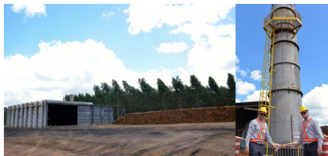
Figure 5. Larger charcoal kiln with 2000 m 3 capacity coupled to with gas incineration (Brazil).
