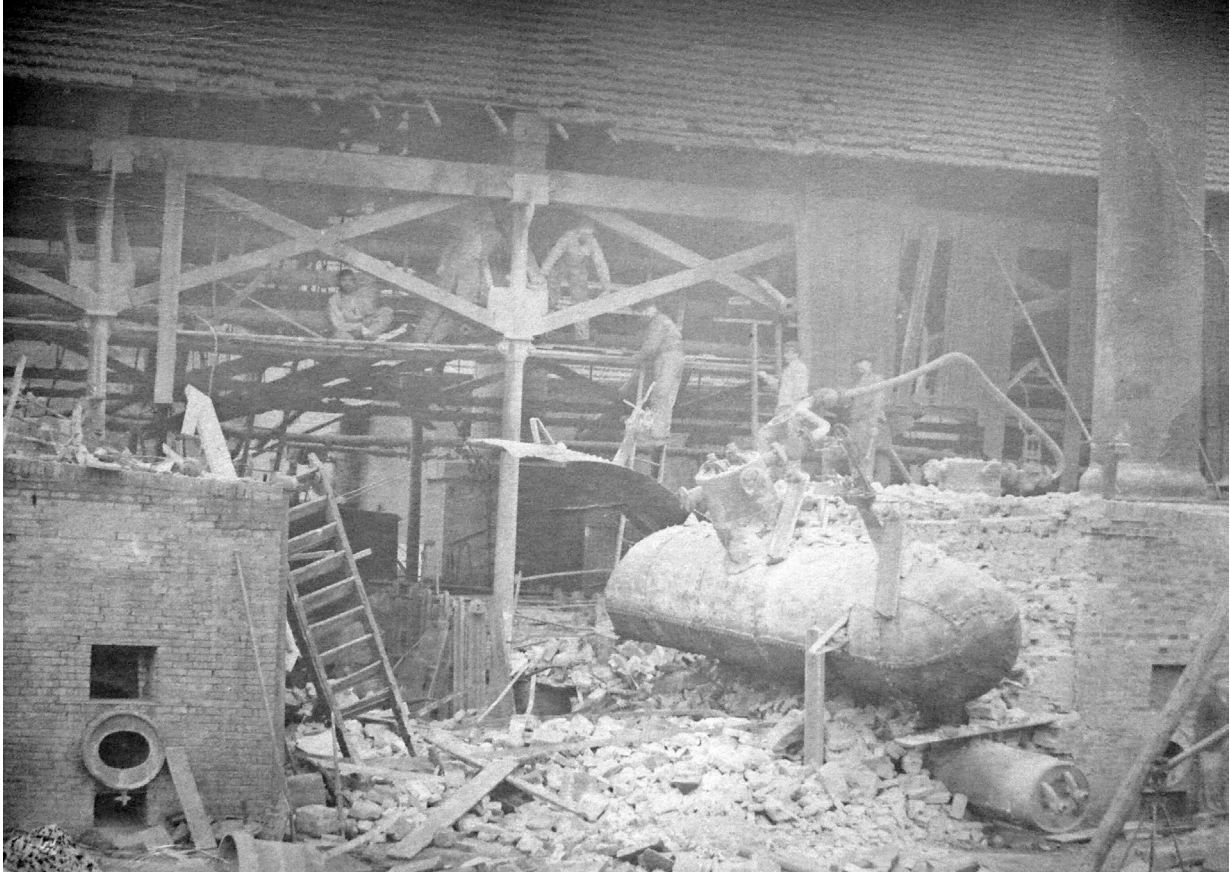
Photo 1. Steam boiler explosions like this one in Paris in 1868 exposed the public to the dangers of industrialization in urban areas
