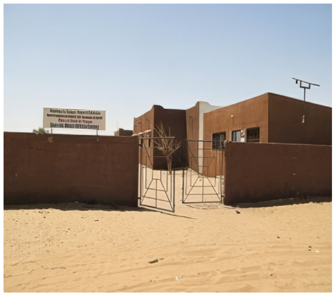
Fig. 4. Infrastructure built after negotiation with an agro-industry.
