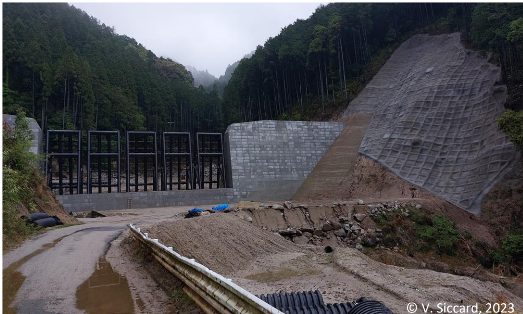
Open check dam: steel frame structure dam
