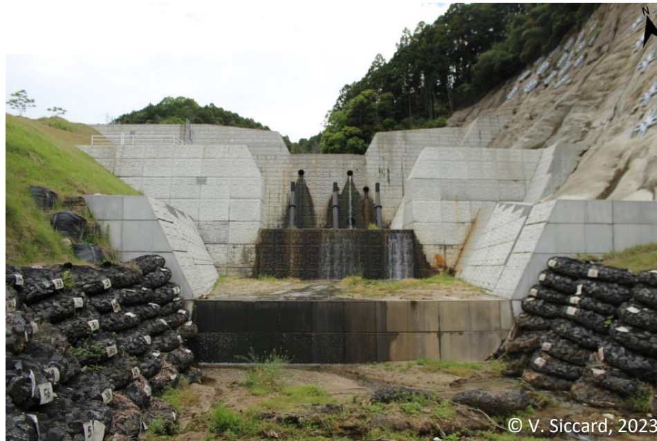
Close check dam: 3 dimensional dam
