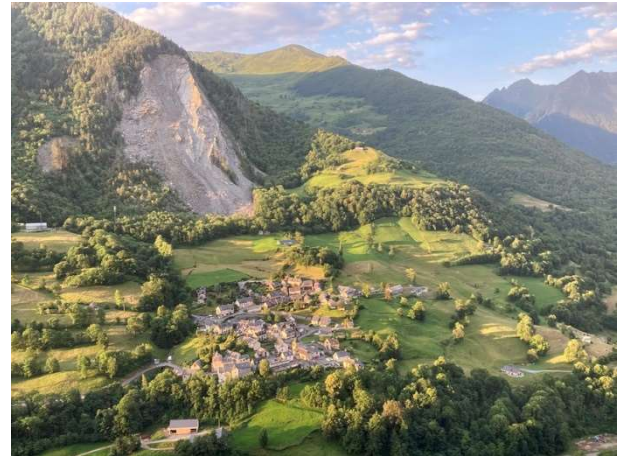
Figure 7. Viella landslide in August 2020 (France)
