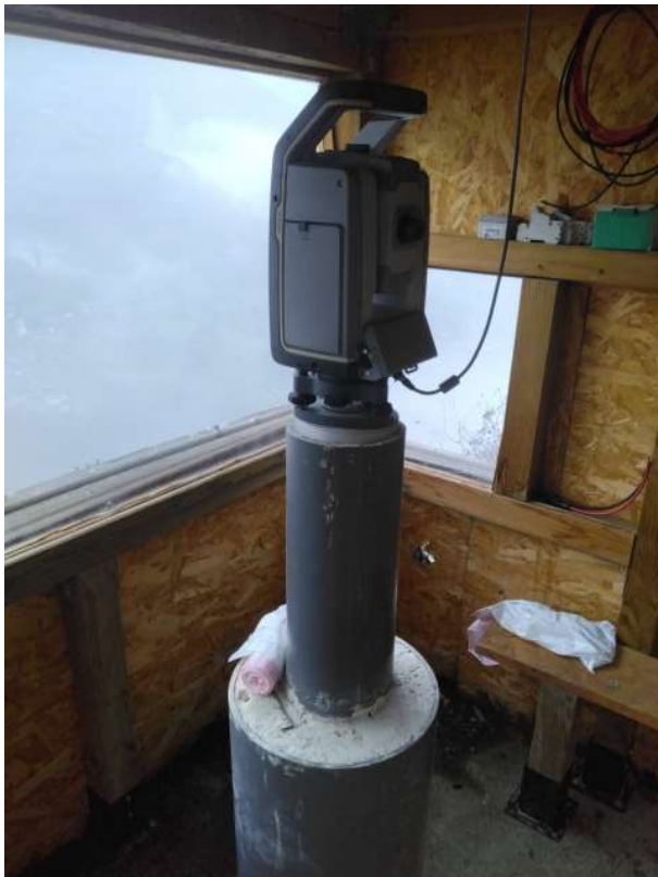
Figure 9. Permanent automated total station Trimble S9 Long Range on the pillar at the monitoring site at Viella landslide (FR)
