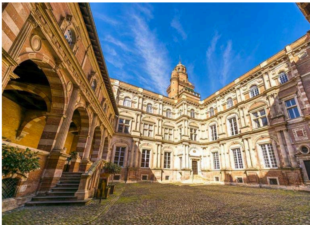
Figure 5. The Hôtel d'Assézat in Toulouse, a building built with the proceeds from the pastel trade (photo: Office du Tourisme de Toulouse).
