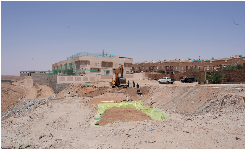
Photo 17. Installation of the pilote waste water treatment plant in Ghardaïa
