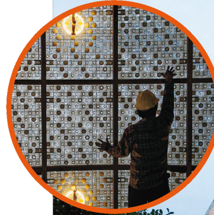
The grooved Polli-Bricks lock together to form panels.
