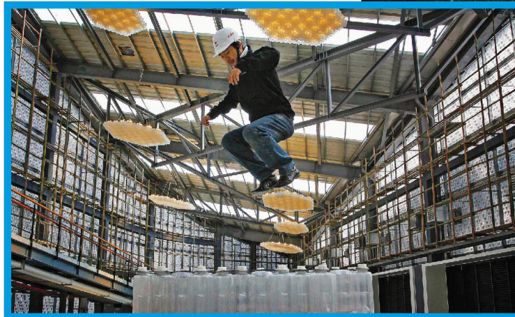
The Polli-Brick panels are lightweight but strong. Huang demonstrates by jumping up and down on them.
