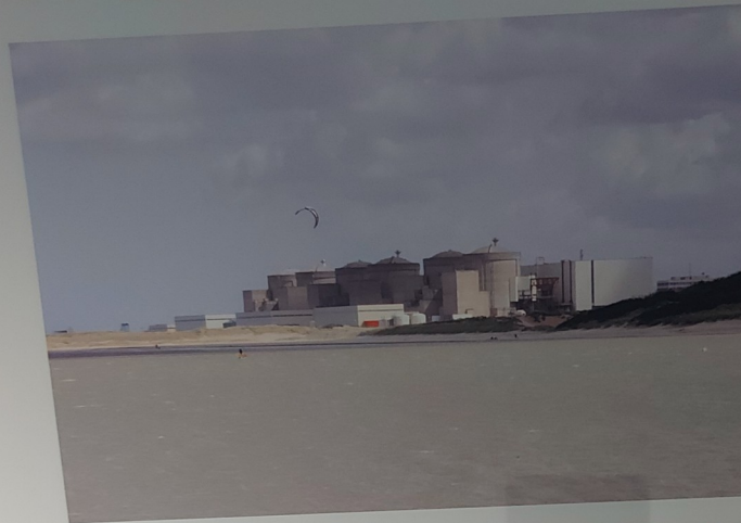
© EDF-CNPE de Gravelines La centrale de Gravelines vue de la mer. Gravelines nuclear plant photographed from the sea.
