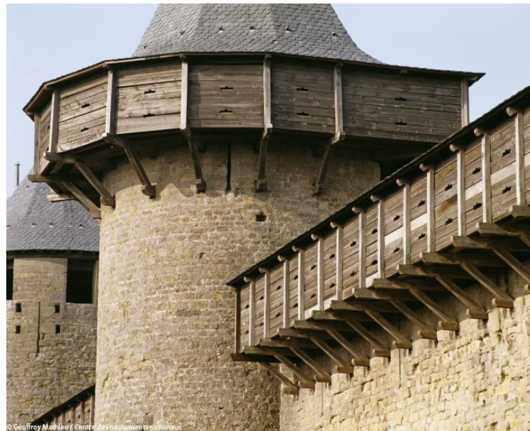
Figure 10. Example of hoarding structures in Carcassonne, France [42].
