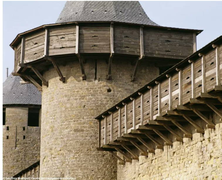
Figure 10. Example of hoarding structures in Carcassonne, France [42].
