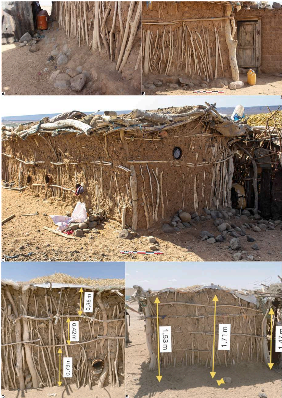
Fig. 4. Wattle-and-daub technique. Foundation and basement with stones and compact mud (A-B). Large pieces of wood are placed vertically at the corners and long sides of the building (B-C). Horizontal poles, unevenly spaced, are then attached to the posts and stakes with cords made of plant materials (D). Stakes of a smaller diameter are placed vertically between these posts (E) – Copyrights: Q. Aubourg, E. Baudouin.
