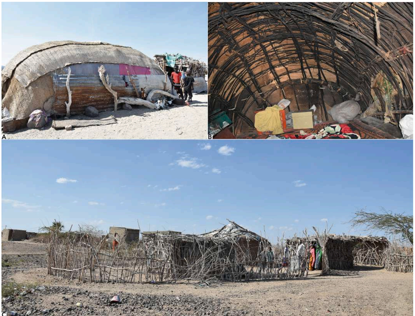
Fig. 8. Traditional light Afar habitat and household organization in Issa. Daboyta covered with basketwork and internal wooden structure (A-B). The Issa inhabited space is enclosed by a hedge of shrubs and thorny plants (C) – Copyrights: Q. Aubourg, E. Baudouin.
