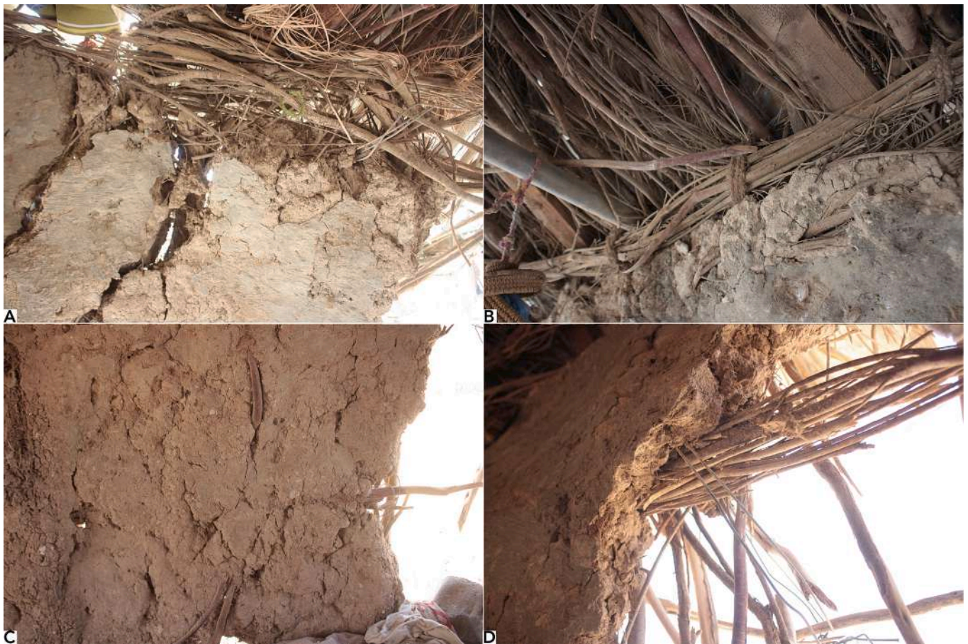
Fig. 5. Wattle-and-daub technique. Poles and branches are attached with cords or fabric rope (A-B). The wet daub is plastered onto the wooden frame and smoothed with the flat of the hand or a tool (C-D) – Copyrights: E. Baudouin.
