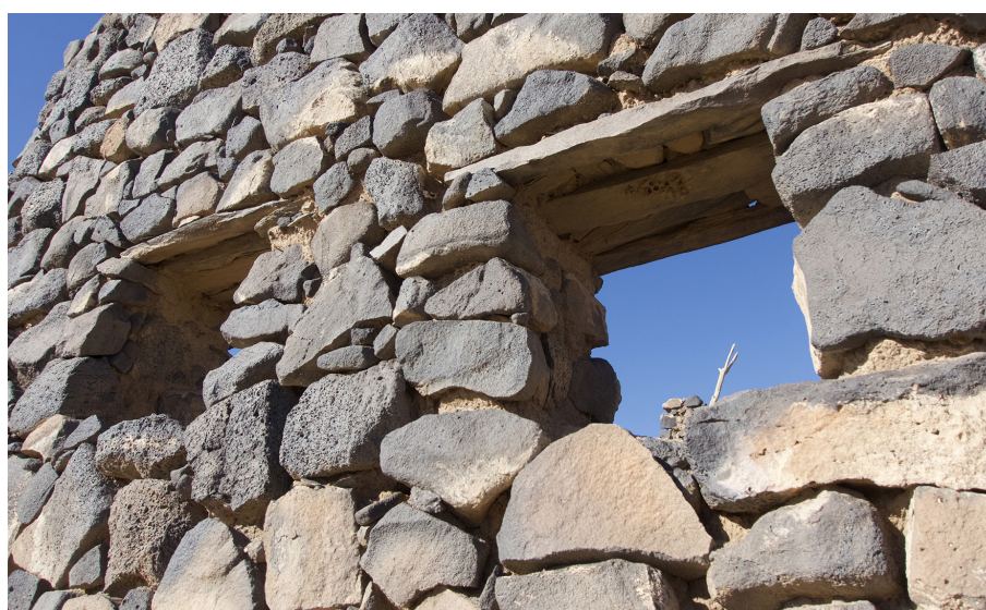
Fig. 21. Green stone used in window lintels. © J. Humbert.
