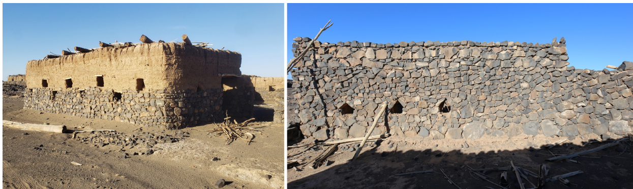
Fig. 7. Two examples of modern houses. The base of the walls, made of basalt stones, is more or less high. Houses entirely built of stone are rare. © E. Laroze.
