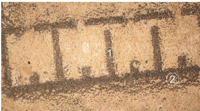
Fig. 10. The remains of UZ006 illustrate the two scenarios described under fig. 9. Inner wall 1 was made exclusively of mud-bricks on a stone base ; outer wall 2 was made of a mixture of mud-bricks and rubble stone, on a stone base. © E. Laroze.
