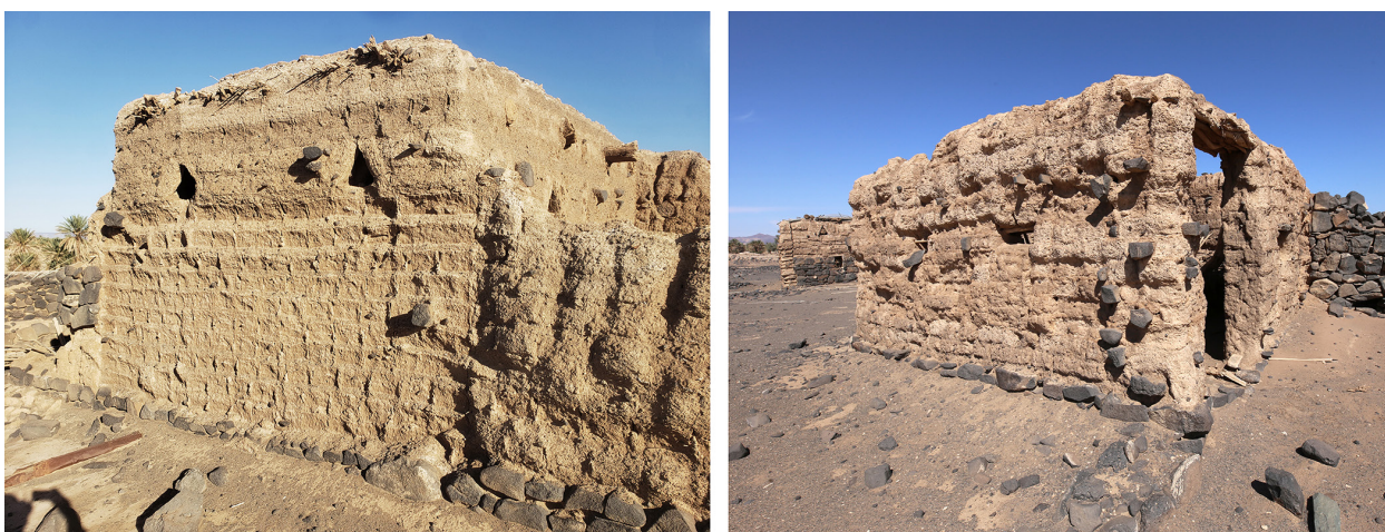
Fig. 6. Two examples of modern mud-brick houses. A varying proportion of basalt rubble may be included in the masonry. The mud-brick walls are laid on a stone foundation. © E. Laroze.
