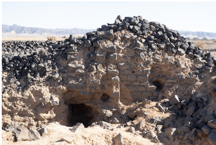
Fig. 18. South face of the preserved northern tower showing, from right to left, the tower, the gate, and the curtain wall. © J. Humbert.
