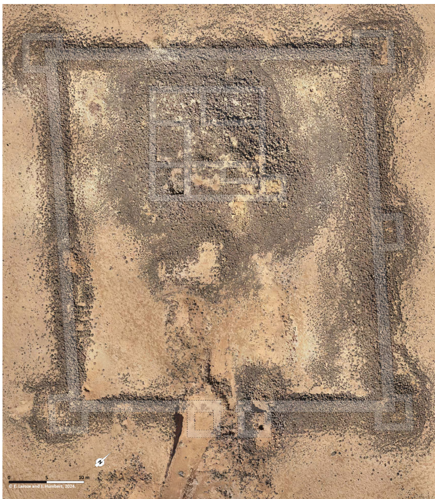
Fig. 13. Orthophotograph and proposed restitution of fort UZ001. © E. Laroze and J. Humbert.
