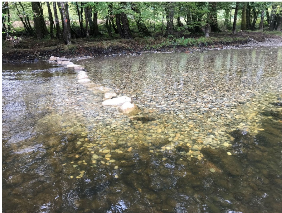
FIGURE 1 | Replenishment for fish spawning in the Dordogne River in 2020. The flow is from right to left. Source: EPIDOR. [Color figure can be viewed at wileyonlinelibrary.com ]
