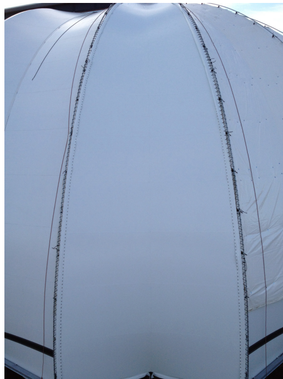
Figure 12 : Three layers are visible: Left inner membrane, Right isolation layer, Centre outer membrane
