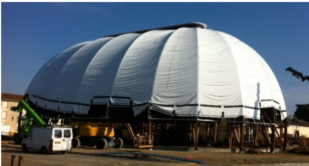
Figure 8 : View of the first layer of membrane
