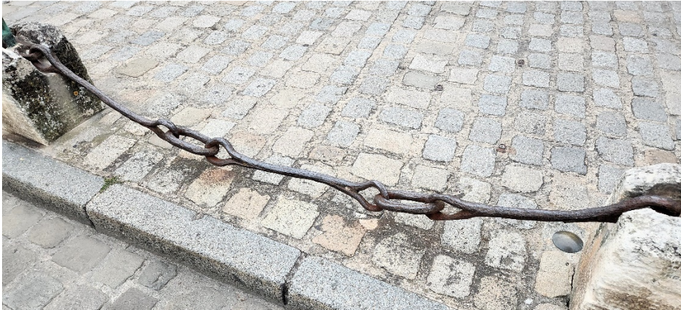
Figure 18. Portion of harbour chain at La Rochelle (France). (Photo de Graauw, 2024)
