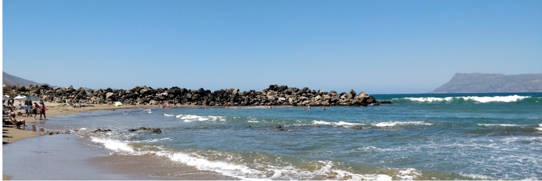
Figure 11. Rubble-mound breakwater at Kissamos (Crete). (Photo de Graauw, 2022)
