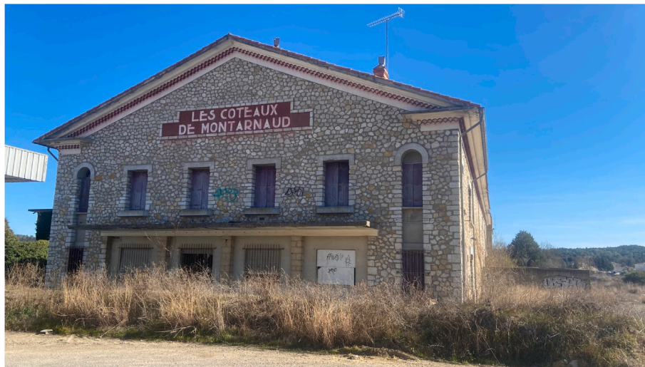
Fig. 2. Cooperative building in Montarnaud, a village located roughly 25 km NW of Montpellier. This cooperative was fused into a much larger, regional cooperative called l'Ormarine. The building lies unused as of this writing. Photo by one of the authors.
