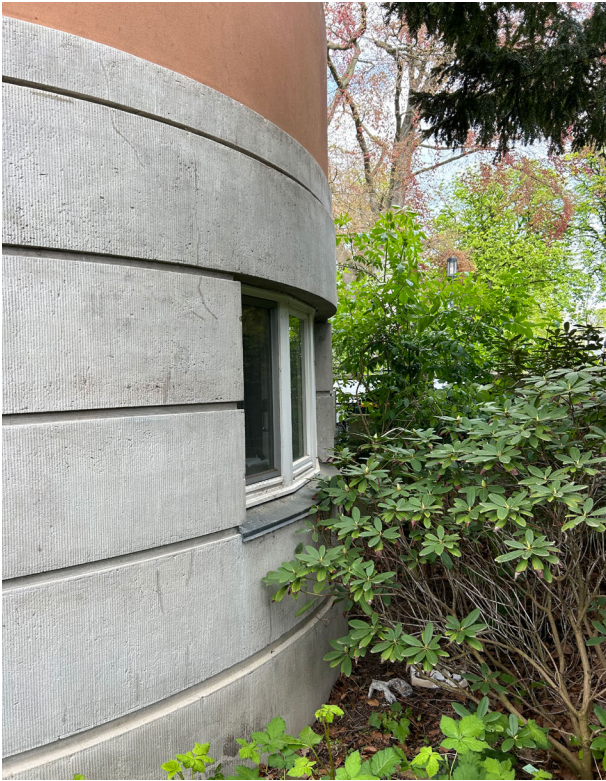
Fig. 2.7.3: Curved wall on eastfacade Ohlendorfsche Villa
