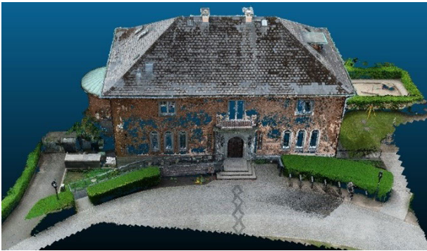
Fig. 1.2.7: Segmented point cloud from photogrammetric image data
