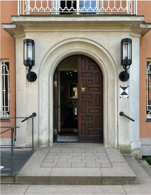
Fig. 2.7.10: Photo documentation, entrance
