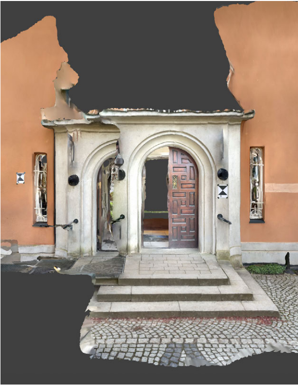
Fig. 2.6.14: Screenshot Scaniverse, misalignment of the entrance portal
