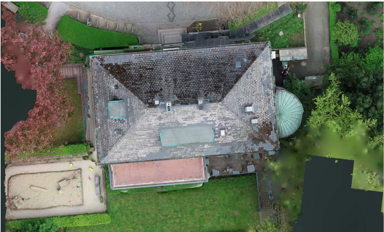
Fig. 2.3.10: Top View Photo taken by a Drone
