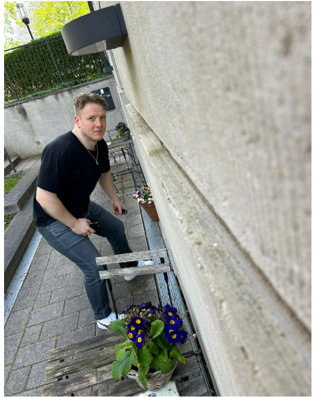
Fig. 2.7.11: Photo documentation, Texture + Material of the westfacade
