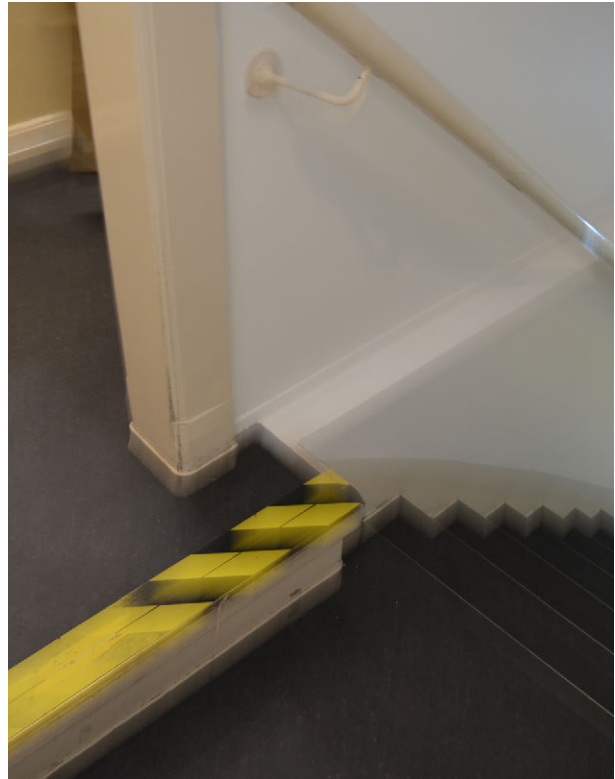
Fig. 2.3.5: Blurred Image of the Staircase to the Basement
