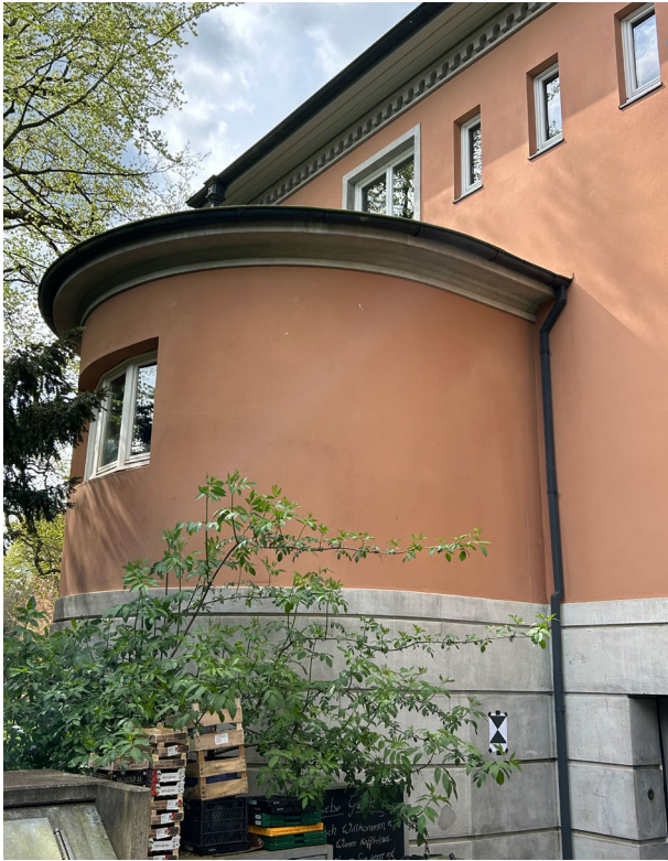
Fig. 2.7.4: Curved wall on eastfacade Ohlendorfsche Villa
