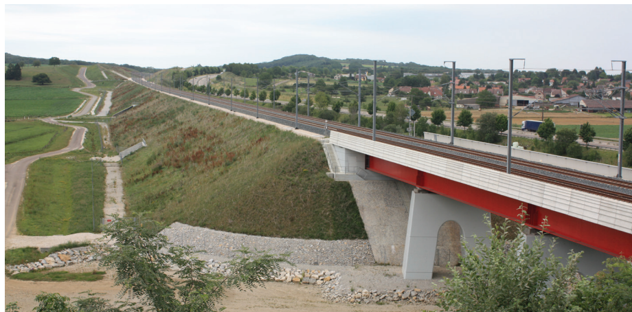
Figure 4. A LGV right-of-way with embankment in a hilly landscape, in the east of France (47.3370°N, 6.0075°E).
