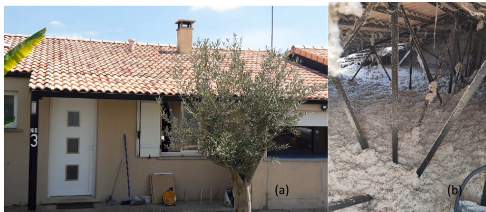
Fig. 2. (a) External and (b) internal views of the studied attic.
