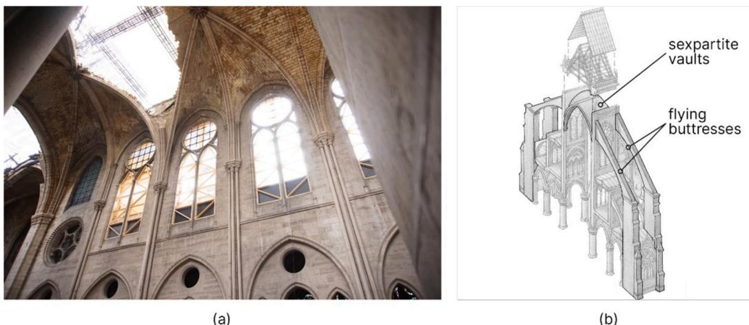
Fig. 1. (a) April 2019 fire damage to Notre-Dame de Paris’ nave and transept vaults (@Bestrema); (b) Notre-Dame choir’s sexpartite vault and buttressing system.
