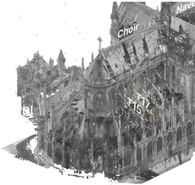
Fig. 6. Location of choir flying buttresses with a crack observed at the head.
