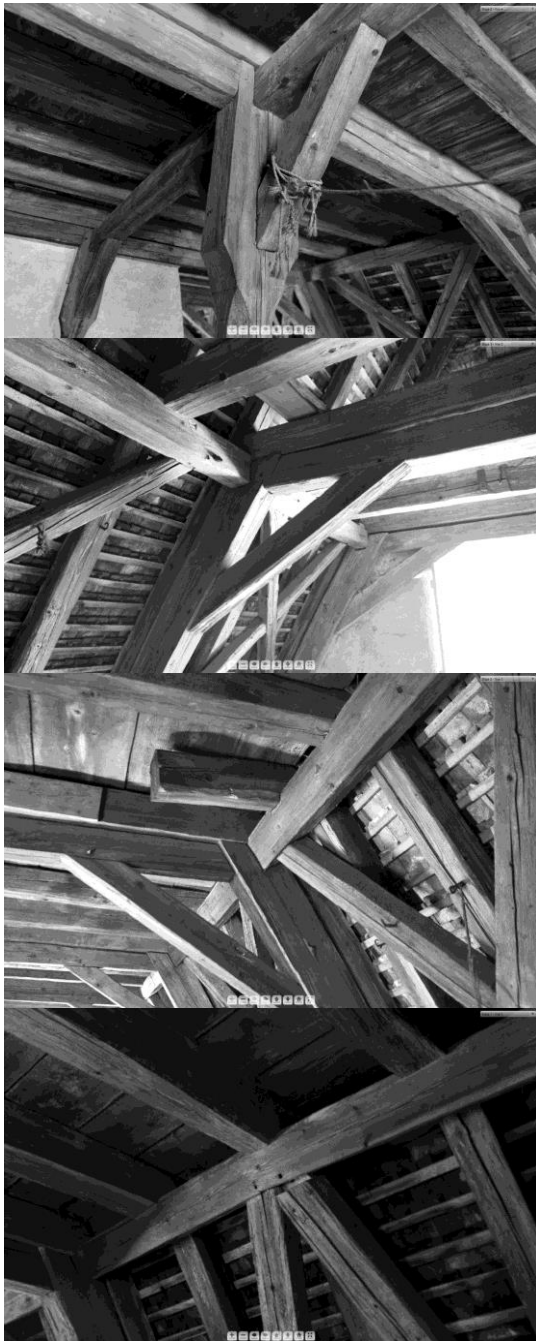
Figure 1.a, b, c: Framework assemblies, d: Assembly deformation
