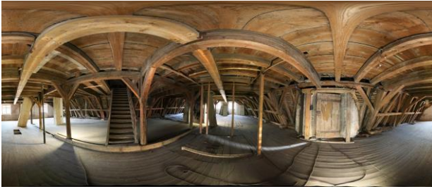
Figure 14: Panoramic view of the first attic level
