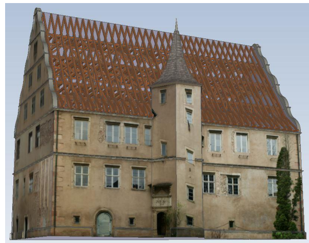
Figure 17: Structured 3D model of the “Seigniory” with accurate model of the wooden framework
