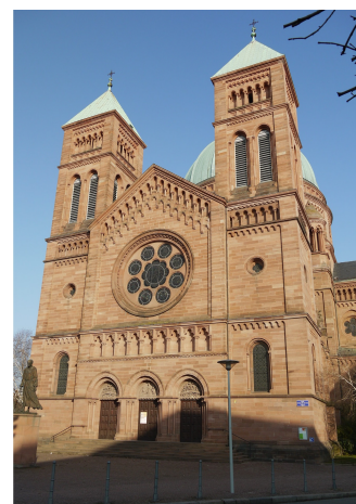
Figure 2. Main facade of the Saint-Pierre-le-Jeune Catholic Church (Strasbourg, France)
