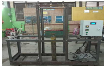
(a) Fabrication of the structural frame
