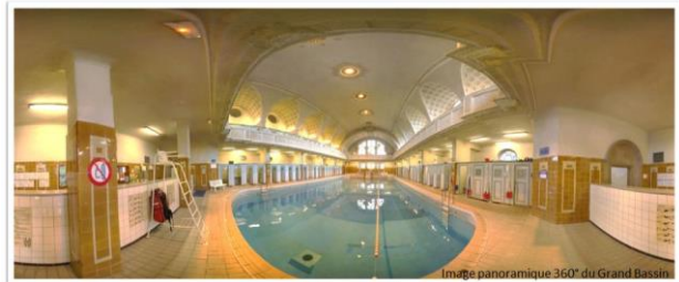
Figure 6 : Panoramic image of the big pool seen from the beach on the north side
