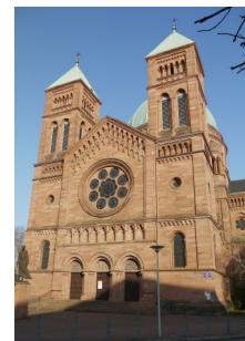
Figure 1. The main façade of the St-Pierre-le-Jeune church, Strasbourg, France built from typical Alsatian red sandstone.
