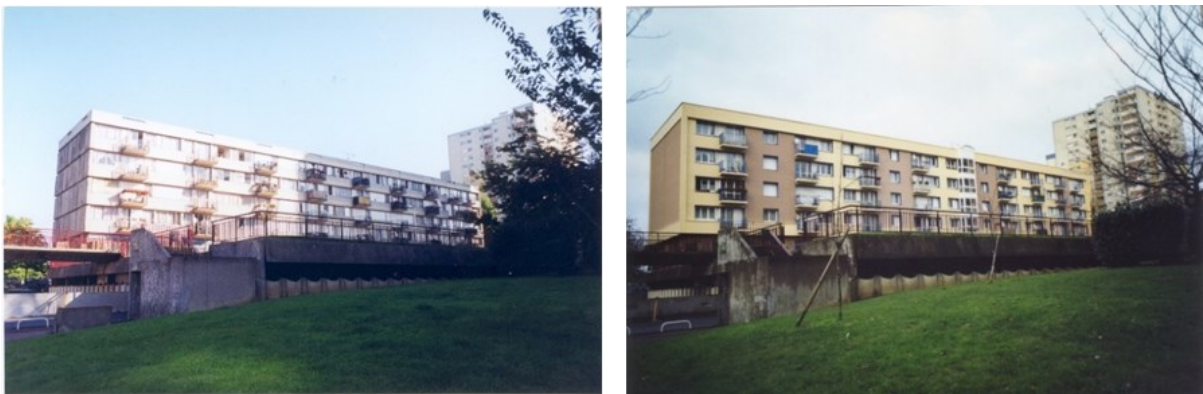
316 Figure 4: Case study building before (left) and after renovation (right)
