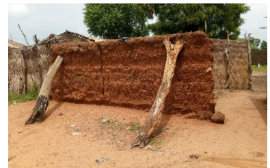
Loss of know-how on how to maintain a bani-bani wall, Wuroahi Community, Fufore, Adamawa State - © UniMaid
