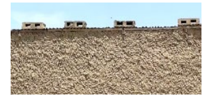
Earth plaster with fingerprints, Dikwa, Borno state - © UniMaid
