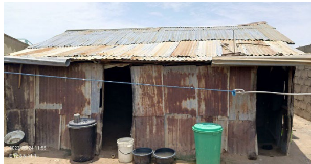
Recycled zinc sheets for roof and walls, Damboa, Borno state © UniMaid
