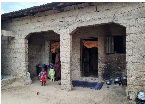
Cement walls, mono-pitch zinc roof, Malakyariri, Borno state © UniMaid
