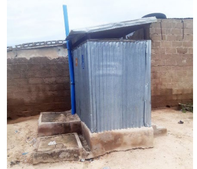
Proper WASH facility in a compound, Shuwari Community, Dikwa, Borno State - © UniMaid
