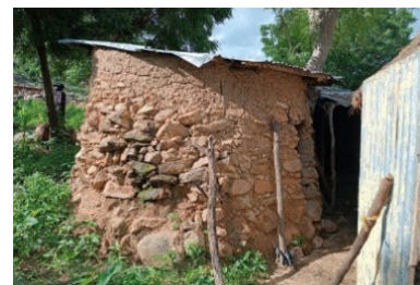
Walls combining stones and earth, Gwoza, Borno state - © UniMaid
