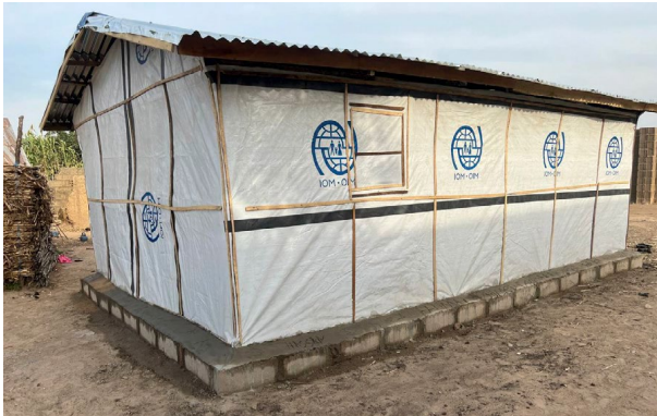
Improved emergency shelter (Dikwa-type) – © IOM
