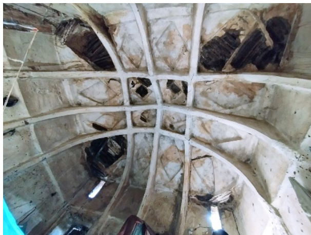
Earth roof with corbelled arches made with azara and plastered with mud mortar and lime (b) in Bade, Gashua, Yobe State - © UniMaid
