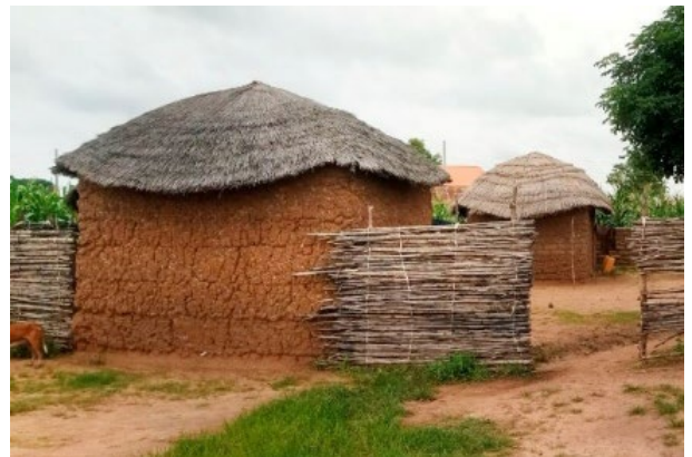
Bani-bani walls and thatch roof, Hong, Adamawa State - © UniMaid
