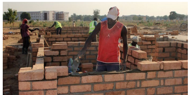
Building with CEB in Maiduguri, Borno state - © IOM Nigeria
