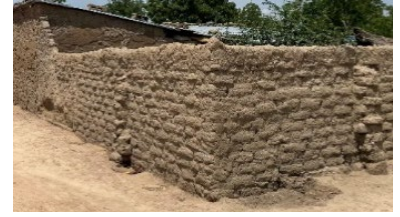
Mud bricks wall, Dikwa, Borno state © UniMaid
