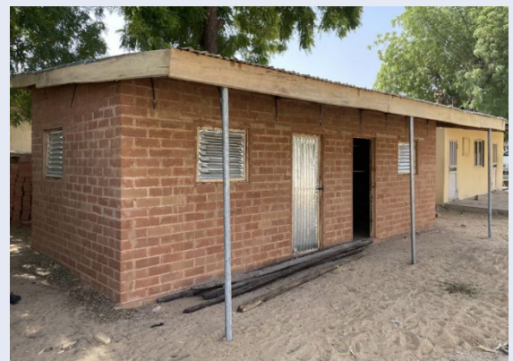
Compressed stabilized durable shelter – © Mercy Corps
