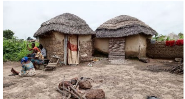
Mud bricks walls and thatch roof, in Hong, Adamawa State © UniMaid
