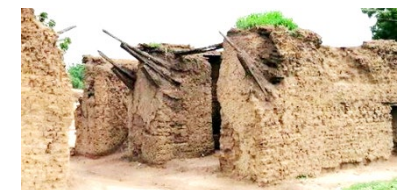
Abandoned earth roof, Rabih house, Ajari community, Dikwa, Borno state - © UniMaid
