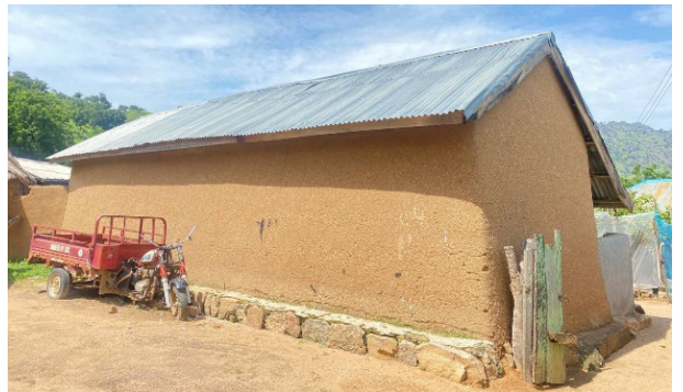
Earth walls and gable zinc roof, Michika, Adamawa State - © UniMaid
