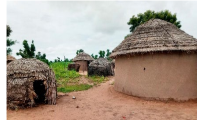
Circular plan shape and thatch roofs, Mbamba, Yola South, Adamawa State - © UniMaid
