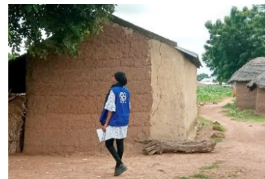
Cement plaster over a bani-bani wall, Hong, Adamawa State - © UniMaid
