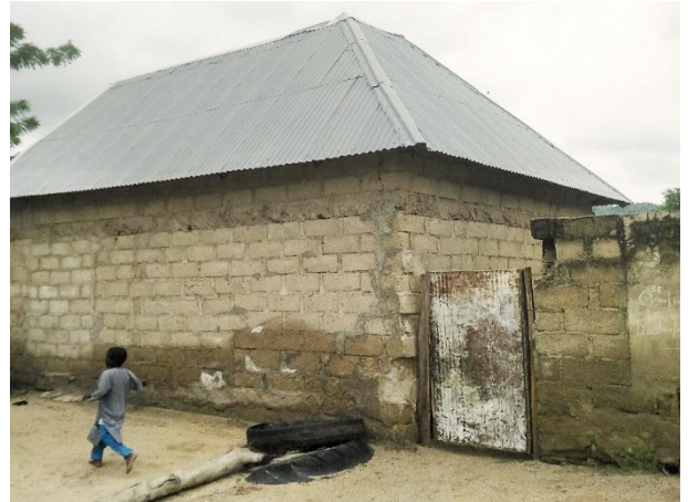
Cement walls and hip zinc roof, Gwoza, Borno state - © UniMaid
