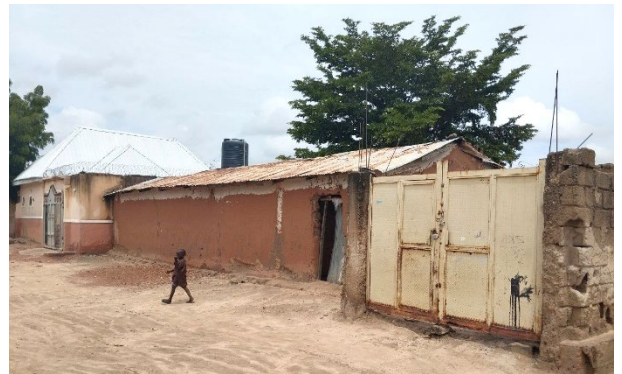
Defensive iron gate, and iron sheets in roofing, Damaturu, Yobe State - © UniMaid
