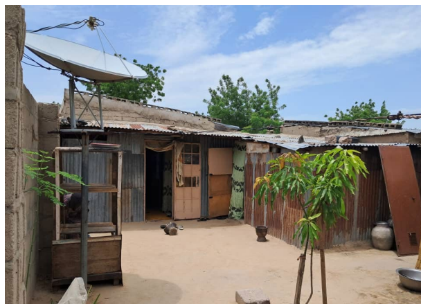
Recycled boards walls, Malakyariri, Borno state - © UniMaid
