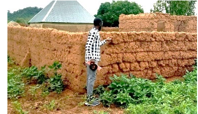
Bani-bani wall under construction, in Gombi, Adamawa state - © UniMaid
