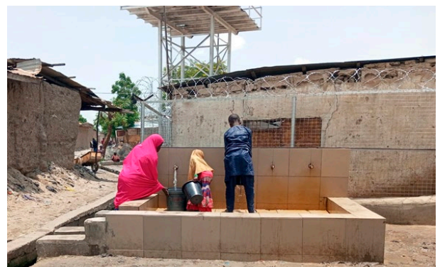
Water tank, community tap and drainage system, Ngala, Borno State © UniMaid
