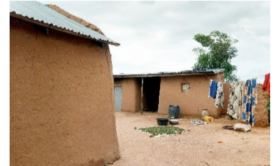
Flexible materials resist ground movements, Gombi, Adamawa State - © UniMaid
