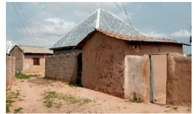
Different roof slopes depending on the material, Fufore-Daware, Adamawa State - © UniMaid
