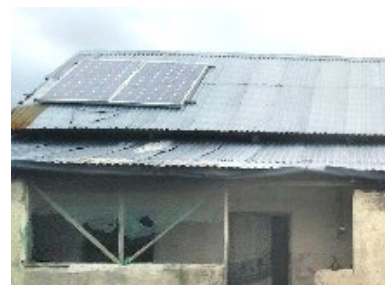
House with solar panels on top of the roof, Gwoza, Borno State - © UniMaid
