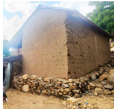
Foundations with stone, Gwoza, Borno state - © UniMaid
