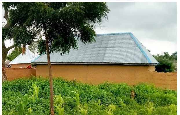
Earth walls and hip zinc roof, Buniyadi, Yobe State - © UniMaid
