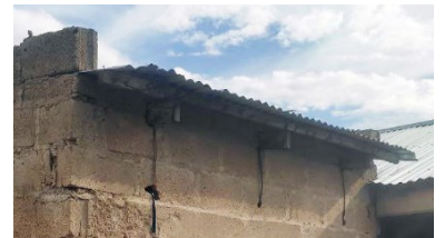
Roof members anchoring ( langa-lang ), Bama, Borno State - © UniMaid
