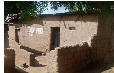
Local construction is still managed in most cases. Here, earth walls and small openings works for a dry and hot climate, Banki, Borno State - © UniMaid
