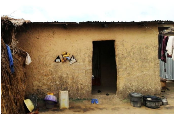
Earth walls and mono-pitch zinc roof, Ajari Community, Dikwa, Borno State - © UniMaid
