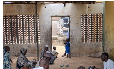
Claustra walls help ventilate indoor spaces, Banki Goniri, Banki, Borno State - © UniMaid
