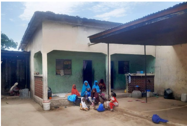
Cement walls, mono-pitch zinc roof, Banki, Borno state - © UniMaid
