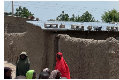
Stones and sandcrete blocks as roof ballast, Bulabulin Community, Dikwa, Borno State - © UniMaid
