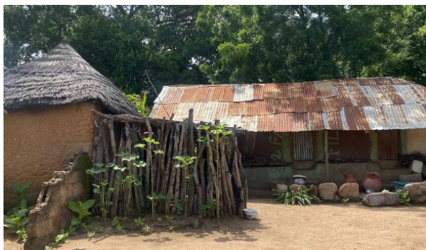
Zinc roofing sheets and thatch covering, Michika, Adamawa state - © UniMaid
