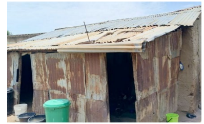
CGI walls and roof for a veranda, Damboa, Borno state - © UniMaid
