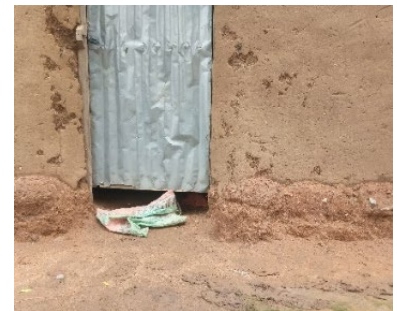
Drained earth footing, Wuroahi Community, Fufore, Adamawa State - © UniMaid
