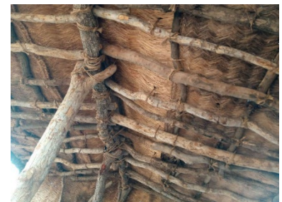
Roof thatch covering a wood structure, Fufore, Adamawa - © UniMaid
