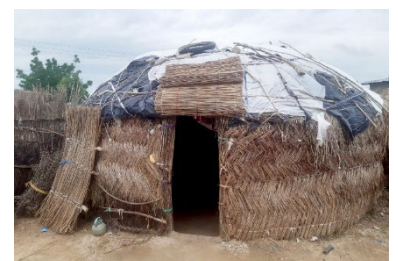
Thatch hut with plastic sheets reinforcement, Dikwa, Borno state - © UniMaid
