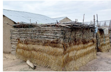
Veranda extension with reeds and thatch, Damboa, Borno State - © UniMaid
