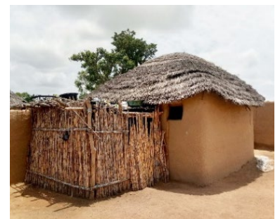
Thatched roof and cornstalk palisade, Gombi, Adamawa state - © UniMaid
