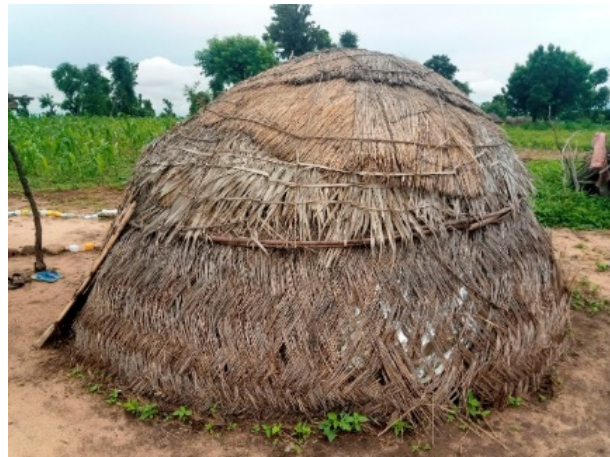
Thatch walls and roof, in Mbamba, Yola South, Adamawa State © UniMaid
