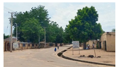
Generous road drainage. Bama, Borno State - © UniMaid
