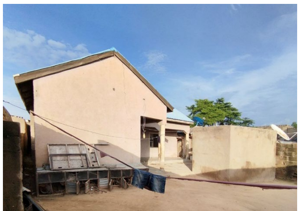
Cement walls and gable zinc roof, Gashua, Yobe state - © UniMaid
