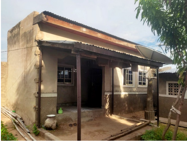
Cement walls, mono-pitch zinc roof, Bama, Borno state - © UniMaid
