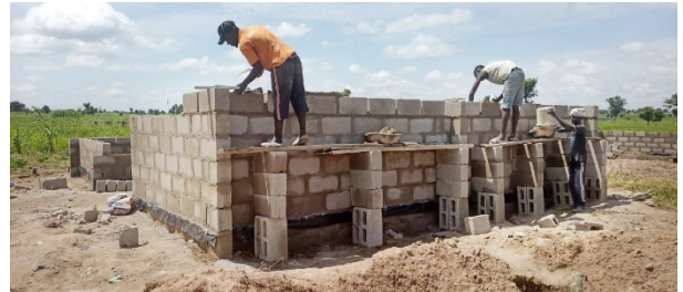
Building with sandcrete blocks in Yola, Adamawa State - © IOM Nigeria
