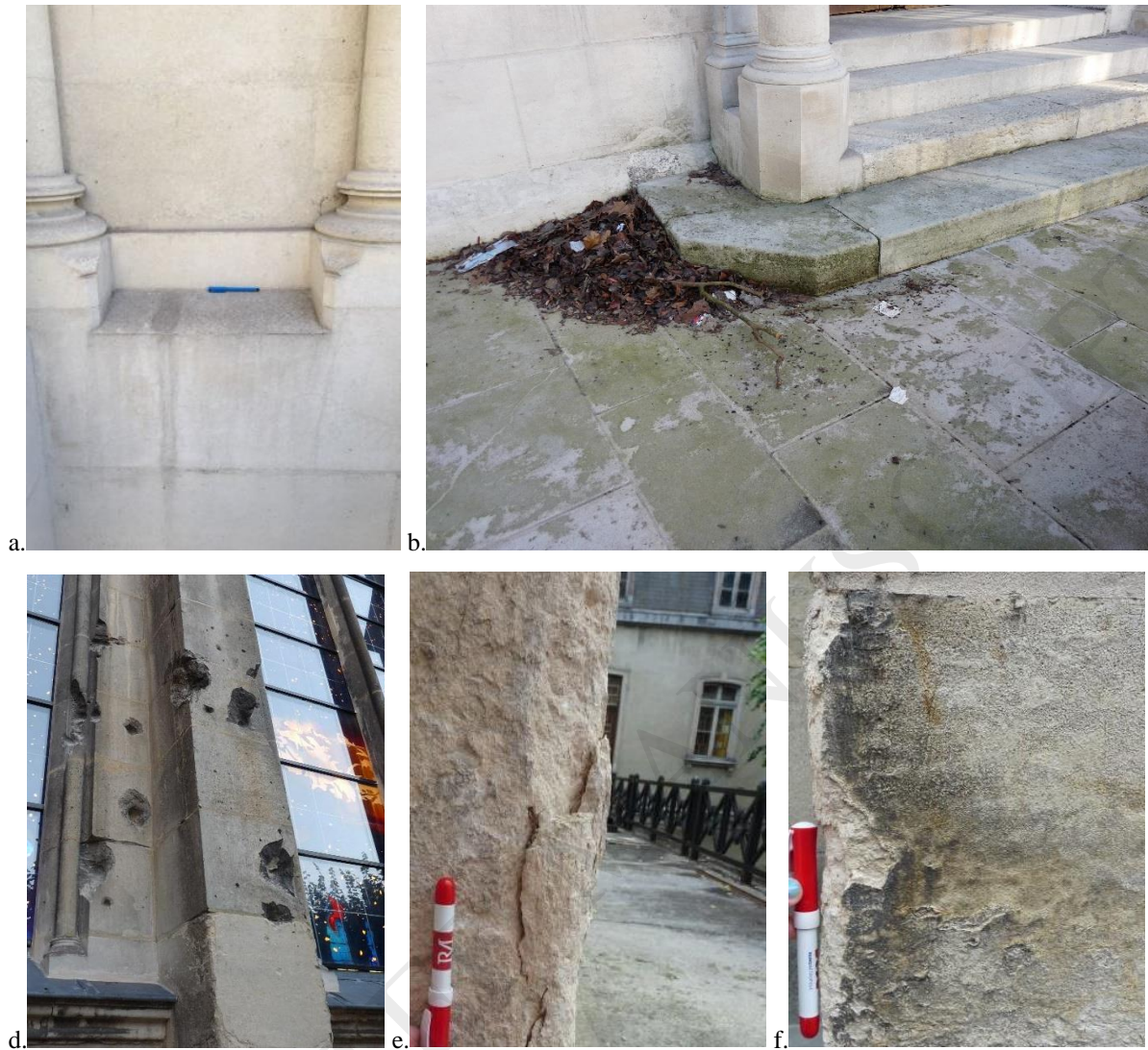
Fig.10 Lower part of an arch (a), floor and stairs (b) of the street façade in June 2016, 4 years after the restoration. Projectile impacts (d), blistering (e,f) and soiling (f) on playground façade in June 2016
