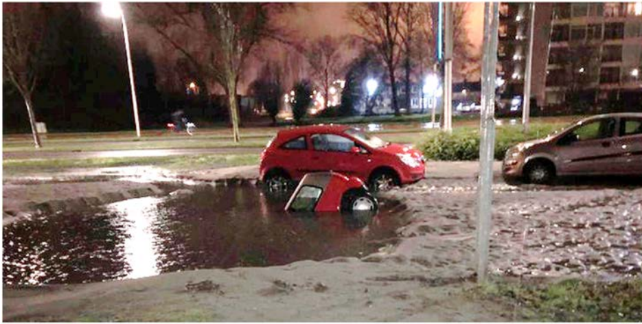
Figure 5.51 Car is completely 'swallowed' in a sink hole that occurred due to a collapse sewer pressure main. (Photo by C. de Haan).
