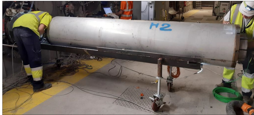
Figure 3. Installation of the thermal source in the HLW demonstrator cell.
