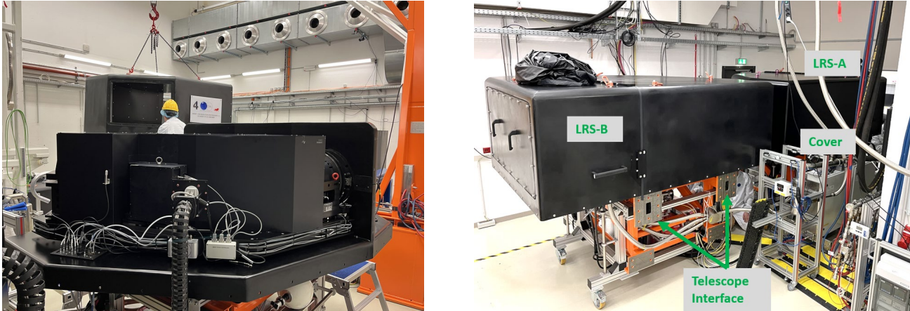
Figure 9: Left: Installation of the Top Cover. Right: Both LRS fully completed with all optical components and with the covers
