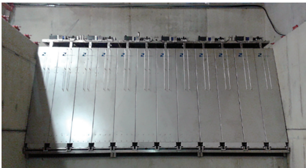
Figure 10. View of the wavemaker after installation
