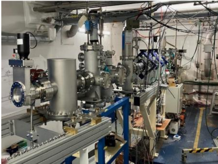
Figure 68: Picture of the assembly of the transport beam line from the SPIRAL 1 facility towards DESIR.
