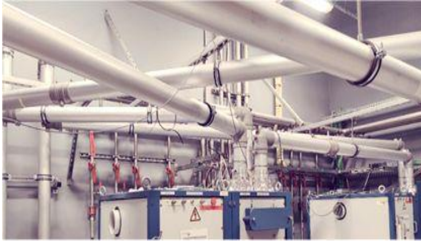
Figure 35: Exemple of RF power distribution
