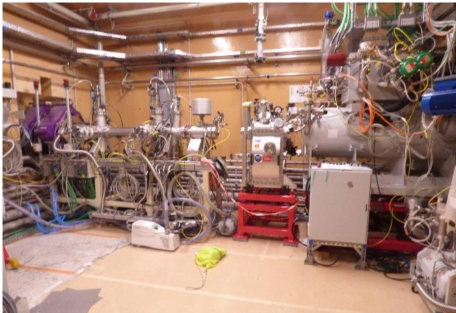
Figure 71: Upstream Beam Line
