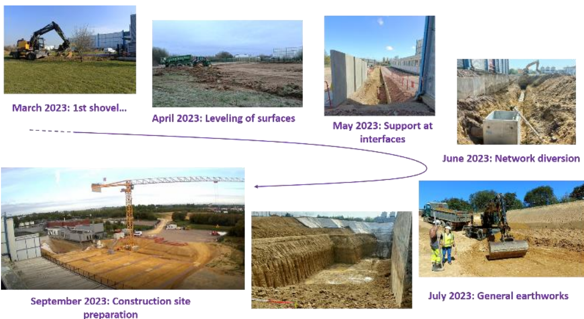
Figure 67: Compilation of pictures of the DESIR construction site preparation in 2023
