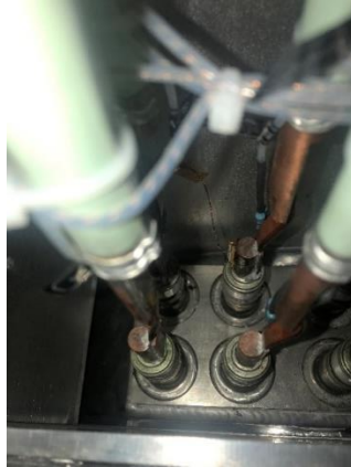
Figure 72: CERNOX temperature monitor on HTS current leads.
