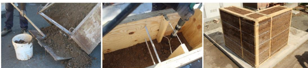
FIGURE 1. Different phases of the construction of the full-scale prototype.
