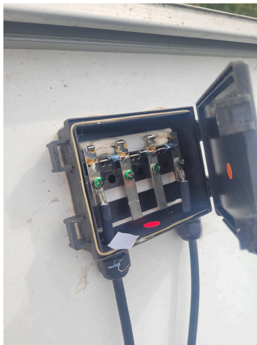
Fig. 3. Bypass Diodes of the PV array.
