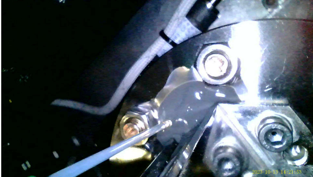
Figure 46: Applying Master Bond EP30-LP epoxy to REB power feedthrough with vacuum leak
