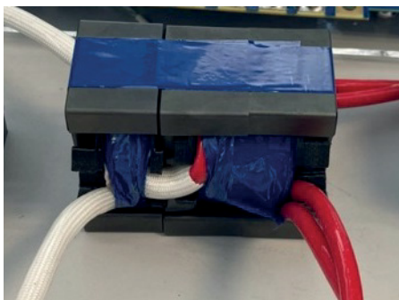
Fig. 6: The experimental realization of the high frequency transformer
