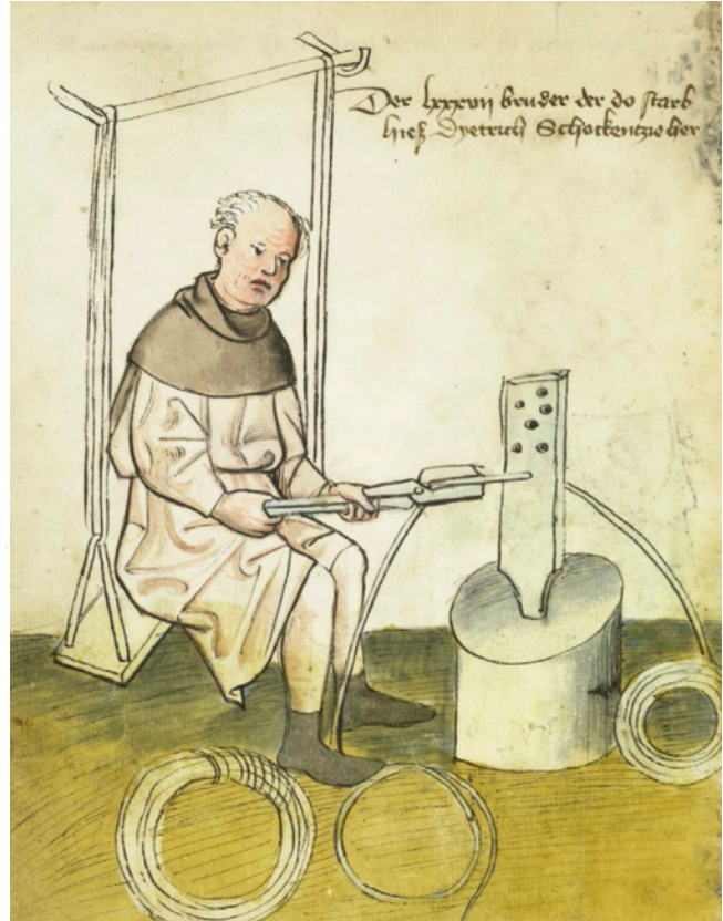
Fig. 6. Medieval wire drawing process [59].
