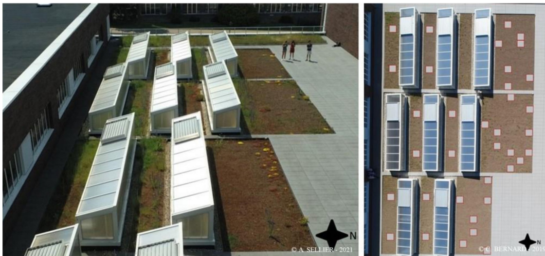
FIGURE 1 The studied extensive green roof and the permanent plots distribution.
