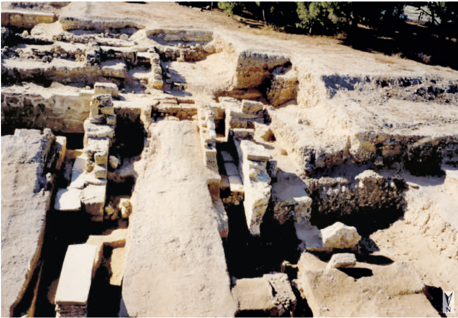
Figure 6 — The last architectural phase in the western part of the shipsheds (© Mission archéologique de Kition).
