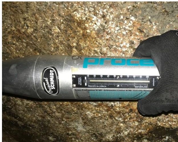
Figure 1. CDG on a tunnel face in Hong Kong and Schmidt hammer test results ( N \approx 0 ).
