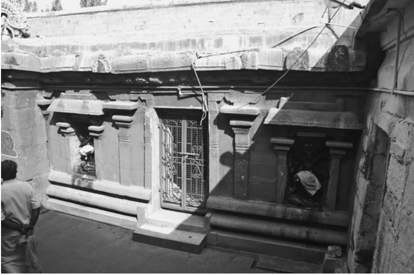
Fig. A.44 Southern façade of the mukha-maṇḍapa of the Tiruvālanturai Mahādeva temple (photo by V. Gillet).
