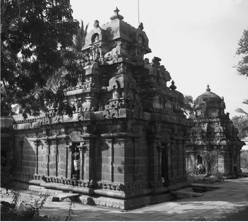
Figure 2.6 General view of the AIM, from the south-east corner (photo by V. Gillet)
