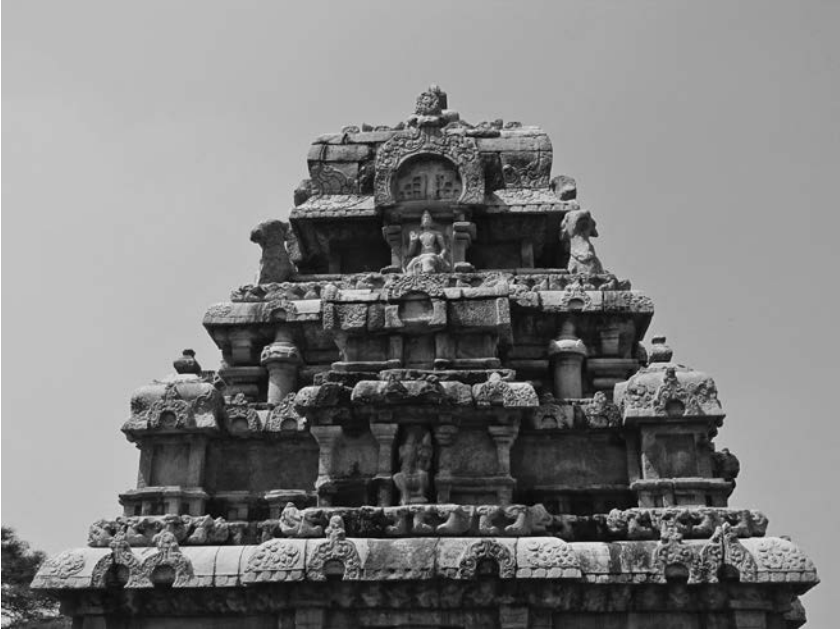
Figure 2.9 Eastern face of the roof of the central shrine of the Müvarköyil (photo by V. Gillet)
