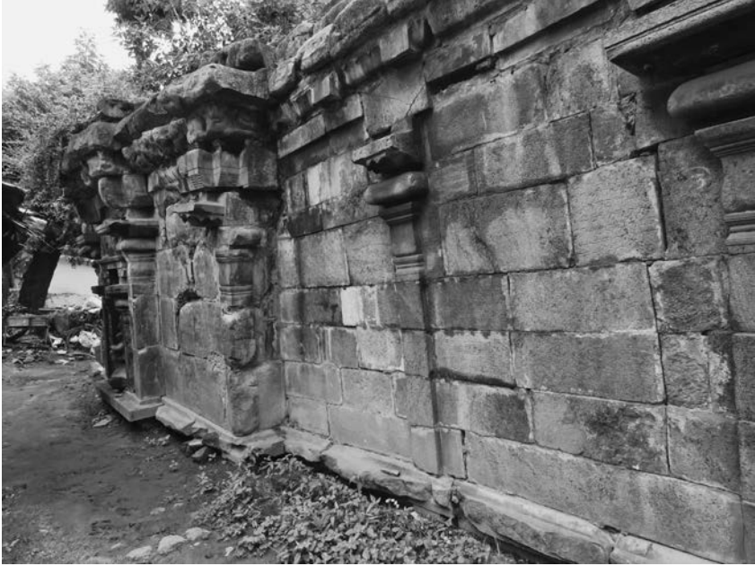
Fig. A.89 Southern side of the Maravanīśvara temple (photo by V. Gillet).
