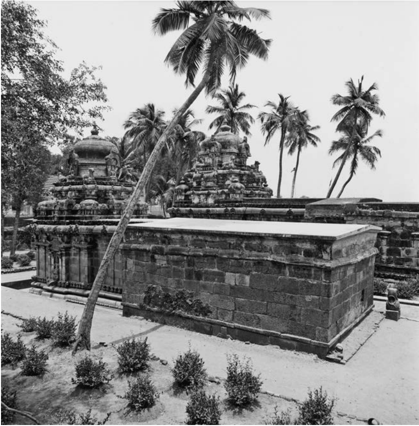
Fig. A.1 General view of the AIM, from the north-west corner (©EFEO/IFP, no. 08332-02, photo by S. Natarajan, 1979)
