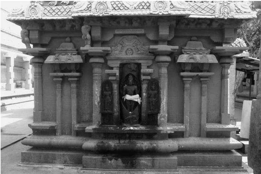
Fig. A.45 Western façade of the sanctuary of the Tiruvālanturai Mahādeva temple (photo by V. Gillet).
