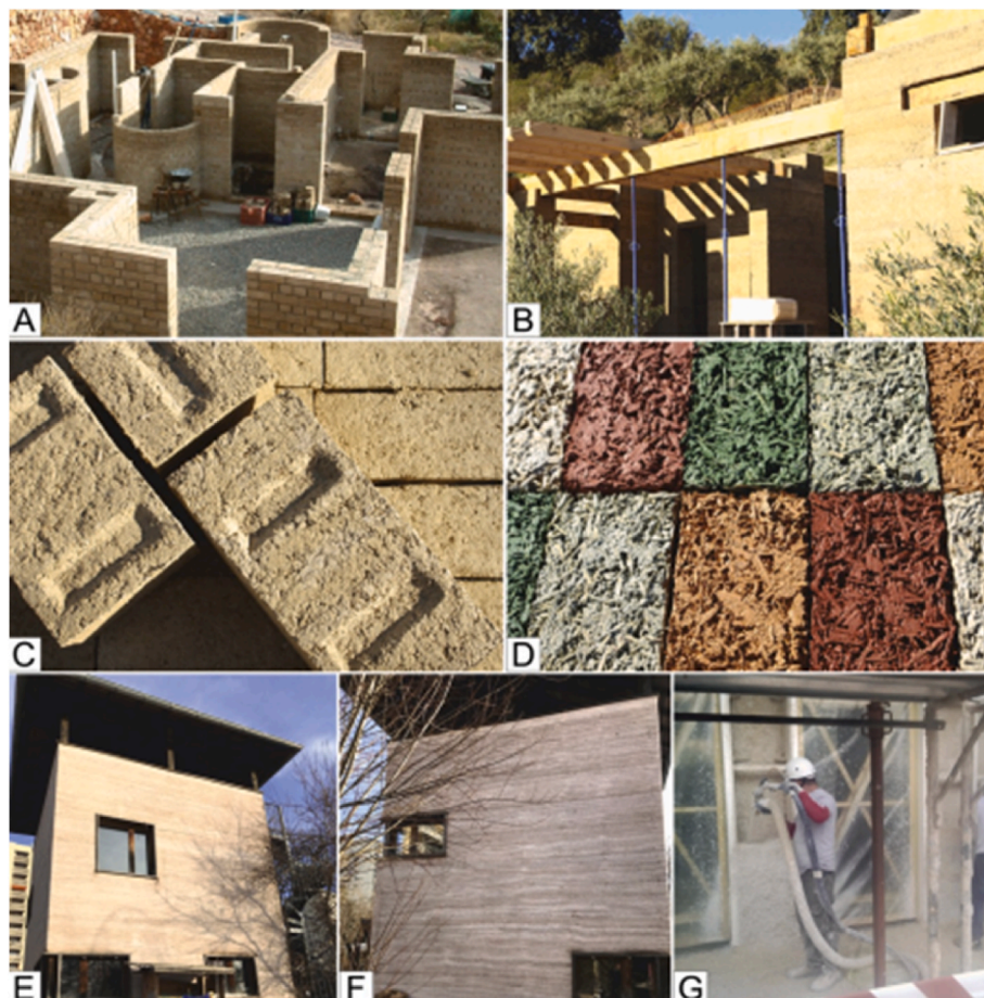
Fig. 27. Hemp concrete constructions can be created using pre-made building blocks (A) or by casting and compacting load-bearing hemp-clay concrete walls (B). These building blocks are made from hemp shives (2–25 mm) combined with either a clay binder (C) or a lime binder, with the optional addition of mineral pigments (D). Images (E) and (F) depict various views of a building constructed with non-load-bearing, cast hemp-lime concrete walls after 20 years of exposure to weather conditions in Switzerland. (G) illustrates the sprayed application of hemp concrete as an exterior coating (Sáez-Pérez et al., 2020).
