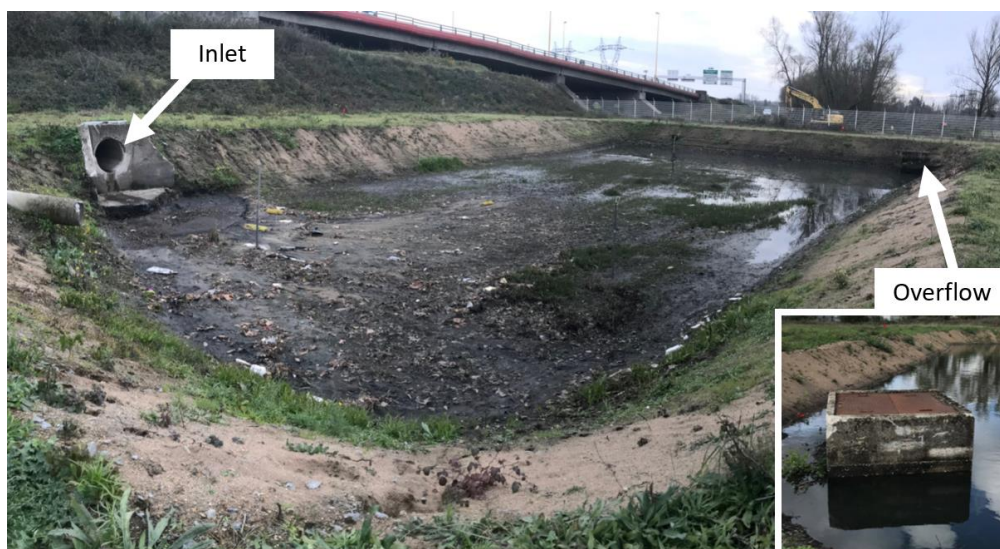
139 Figure 1: Photograph of the studied infiltration pond. The inlet is located on the left side of 140 the pond. A close-up of the overflow is shown in the bottom right corner.
