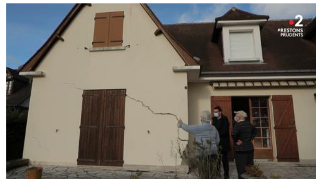
cracked house in the commune of Cour-Cheverny not recognised as a cat-nat drought since 2018 (CEREMA)
