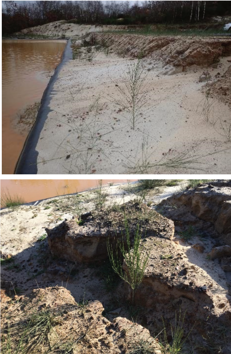
Figure 6 Intensive erosion of tailings in case study 2
