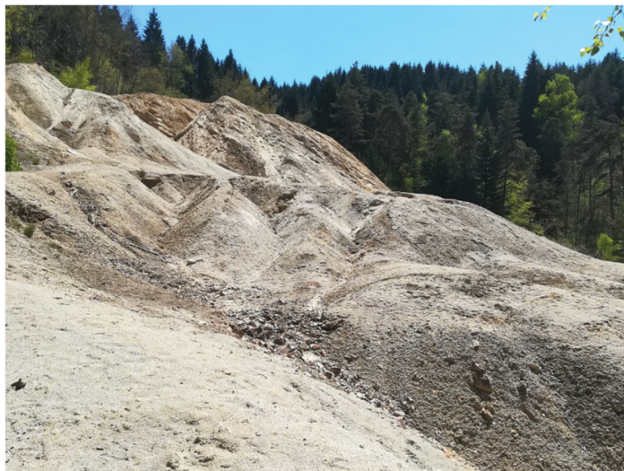
Figure 1 Example of highly eroded tailing deposit in a semi-mountainous region (case study 1, France)
