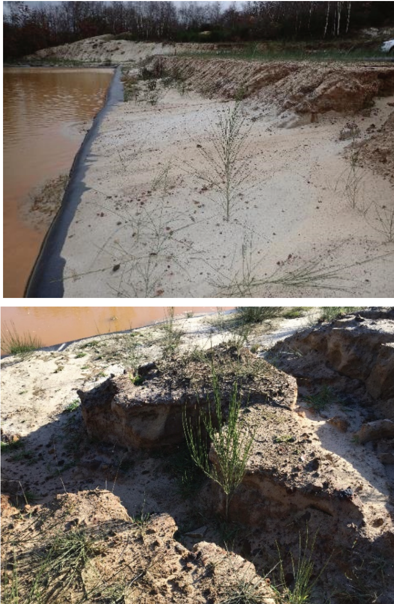
Figure 6 Intensive erosion of tailings in case study 2
