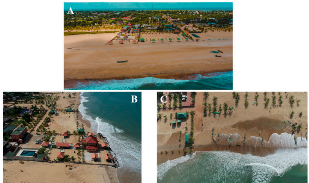
Figure 10. The imagery of beach resorts affected by ECWLs; (A) an aerial view of two major beach resorts (Aborigines beach resort and Agblor Lodge) in Keta without flooding; (B) gradual flooding of the Agblor Lodge and Aborigines beach resort being affected by ECWLs; (C) an aerial view of wave overtopping in the Keta area due to ECWLs. (Photo A obtained from https://www.agblorlodge.com/gallery_cat/aerial-photograph/ (accessed on 21 April 2023); photo credit of B and C: Brempong Emmanuel).
